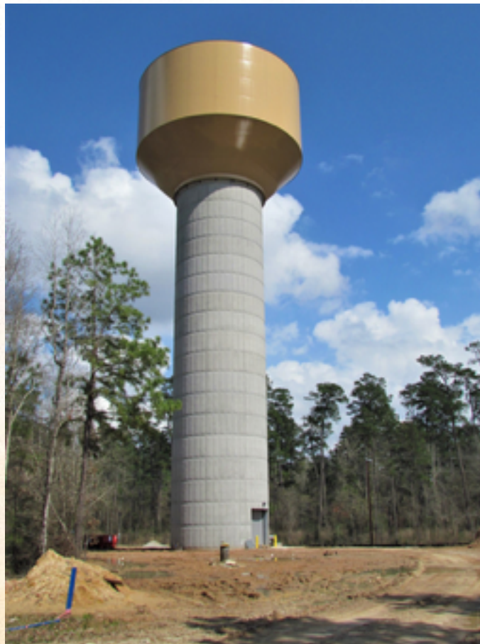
Figure 1: MSEC Water Tower
